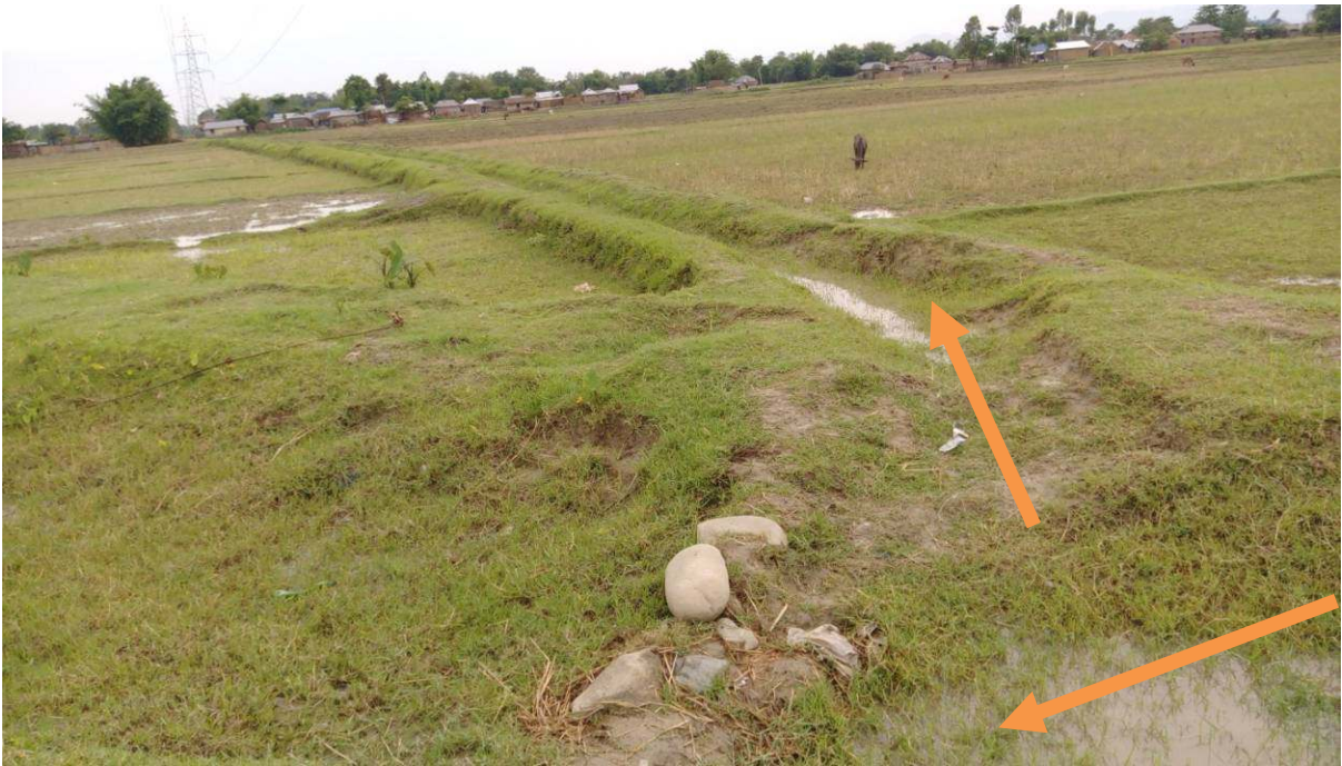
Pic.9: S10-T4, (Ch. 0+655), Masonry structure and unit outlet of WC4R are
