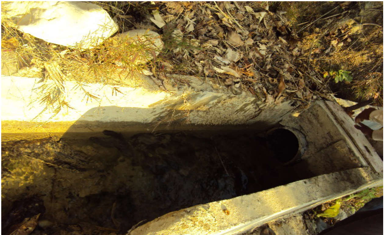
Figure 4: Iron trash rack to be provided in front of Pipe to protect the chance of blocked inside pipe canal.
