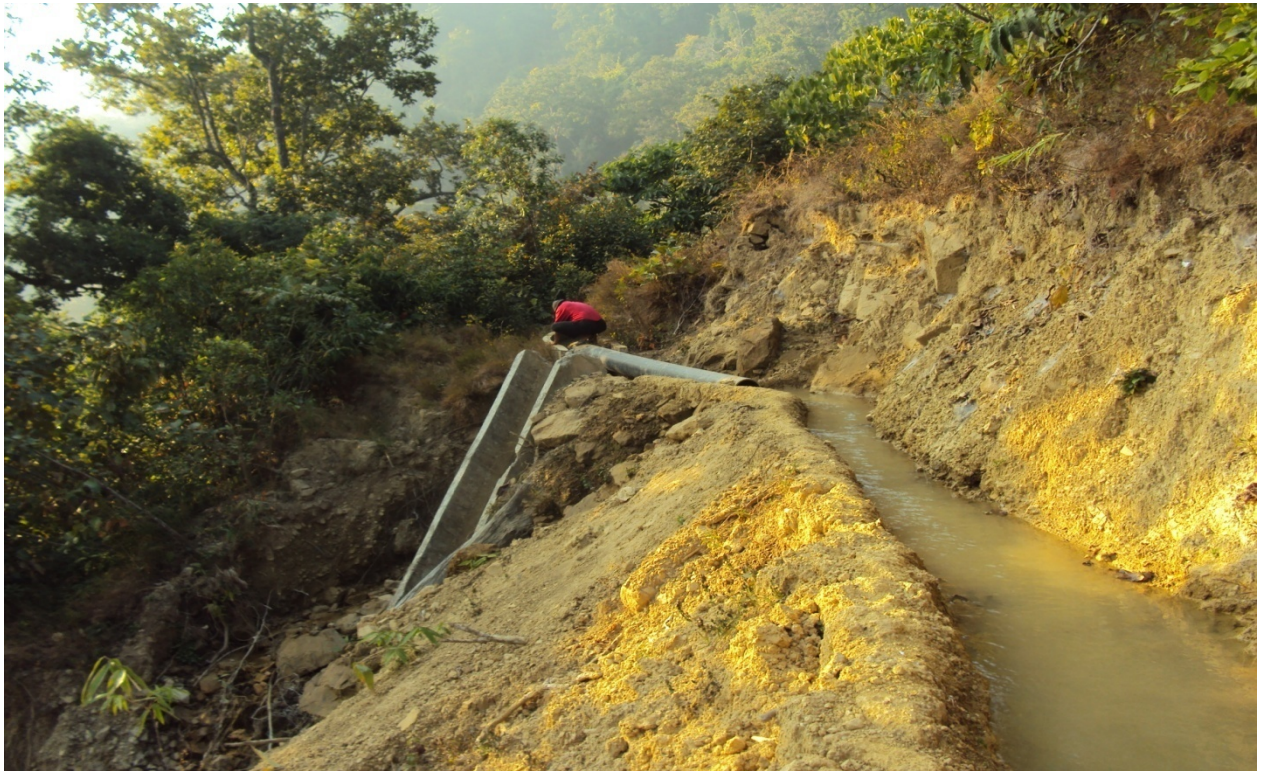
Figure 5: Earthquake effect on main canal on right side broken piece of RCC lined canal of 190 m length.
