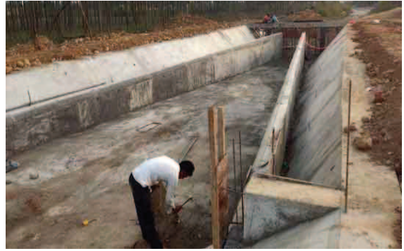
LCW being constructed at Gyani
