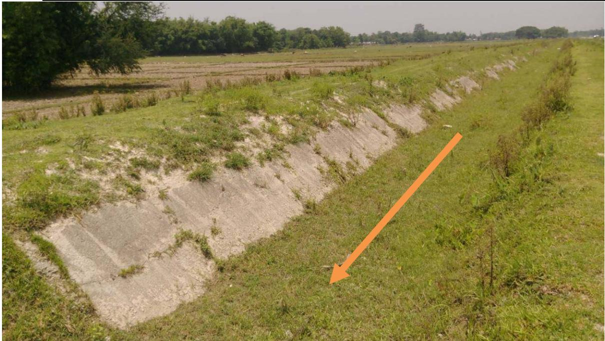
Pic.4: S10-T6, (Ch. 0+570), damaged lining due to vegetation growth
