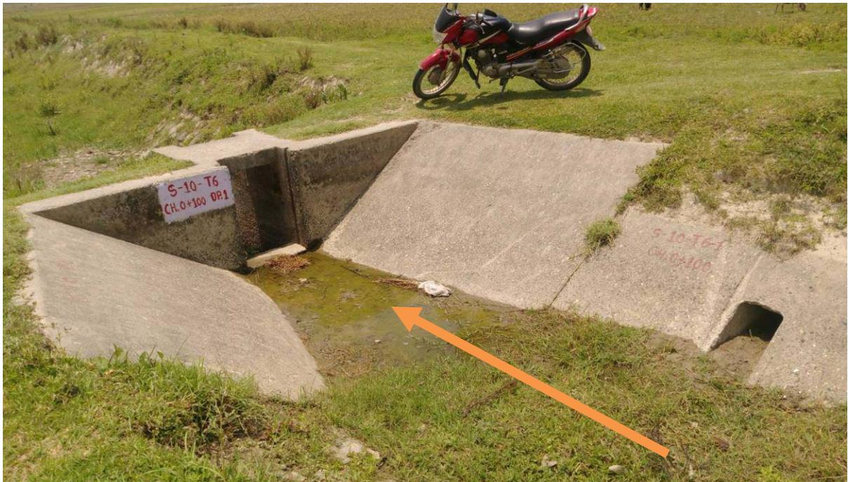
Pic.3: S10-T6, (Ch 0+124), About 10 cm depth of silt deposited at u/s side of
