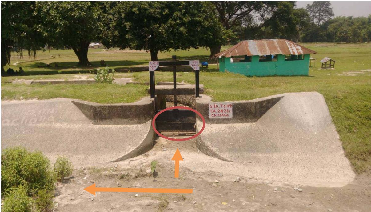
Pic.1: S10-T6, (Ch.0+000), Corrosion on gate plate and holes on bracing frame of HR1
