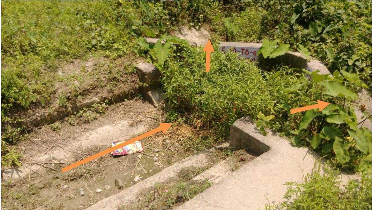
Pic.9: S10-T6, (Ch. 2+231), about 40 cm depth of silt deposited and vegetation growth
