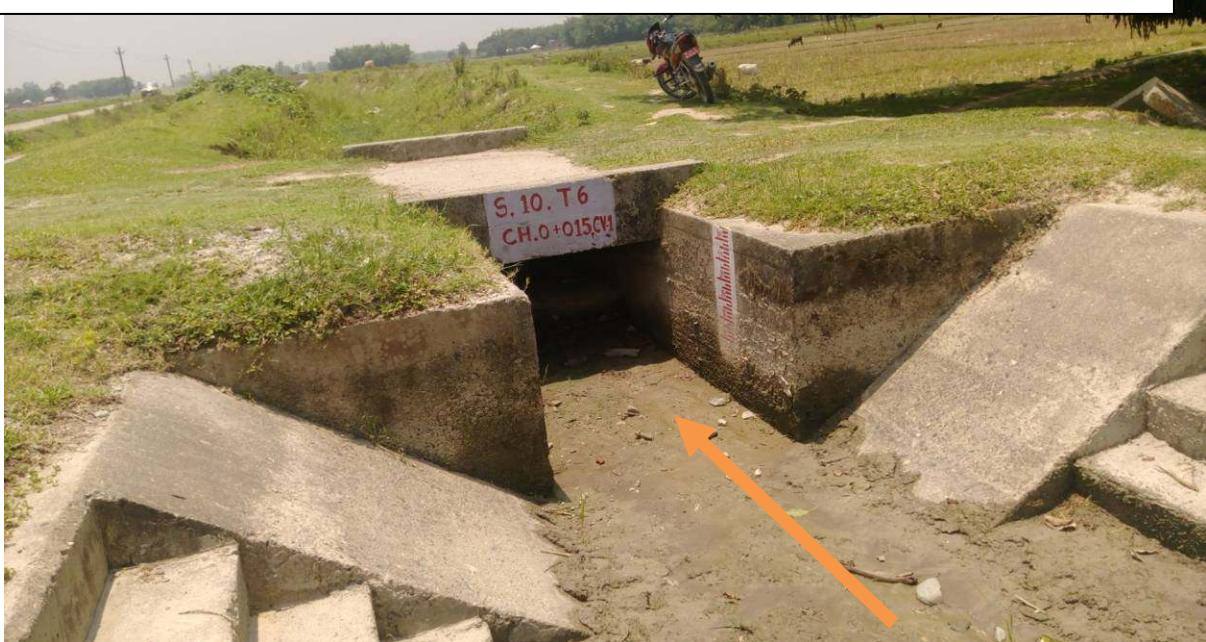
Pic.2: S10-T6, (Ch. 0+015), About 10 cm depth of silt deposited at u/s side of
