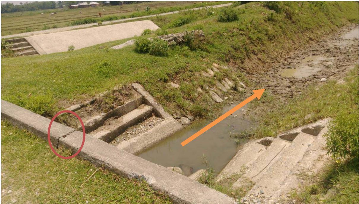
Pic.5:S10-T6, (Ch. 0+677), About 20 cm depth of silt deposited and vegetation growth at u/s and d/s and d/s wall of PCV1 is cracked
