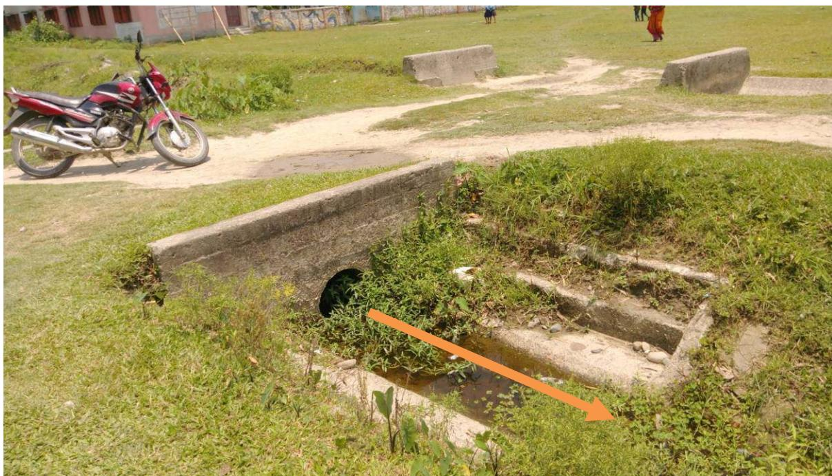
Pic.7: S10-T6, (Ch. 1+755), About 20 cm depth of debris deposited at u/s side and vegetation growth at the d/s side of PCV3
