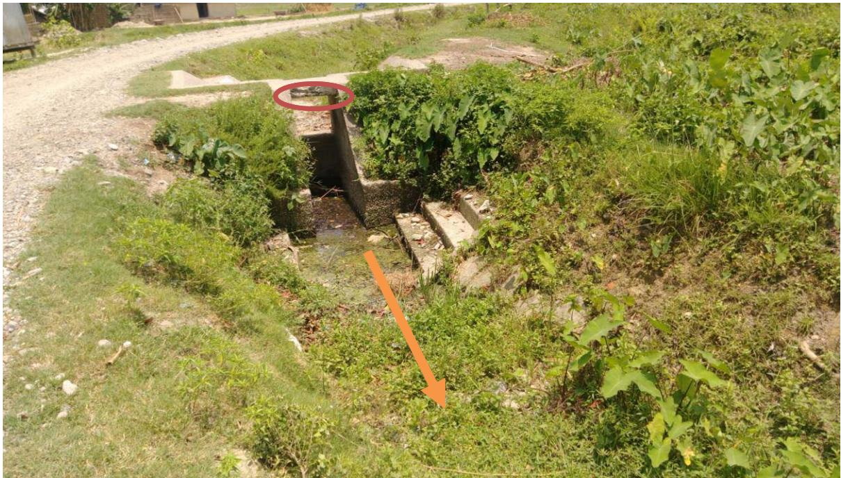
Pic.6: S10-T6, (Ch. 1+605), About 20 cm depth of silt deposited and vegetation growth at d/s side of DP2 and spalling and cracked deck slab
