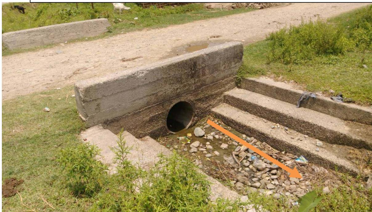
Pic.8: S10-T6, (Ch. 2+215), About 20 cm depth of debris deposited at u/s side and stone deposited at the d/s side of PCV4
