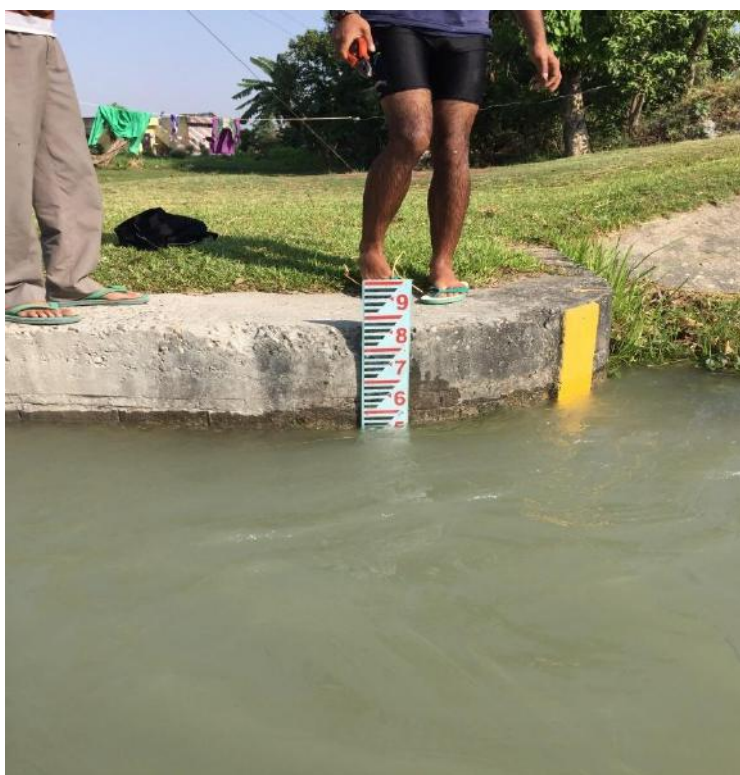
Fig: Installation of Gauge at Flume
