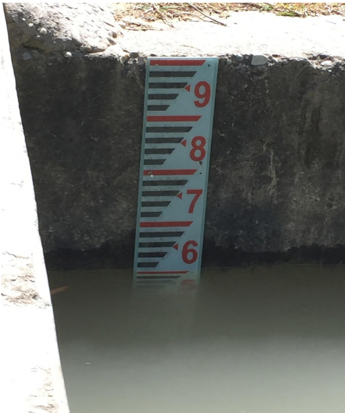
Fig: Installation of Gauge at drop of suda branch
