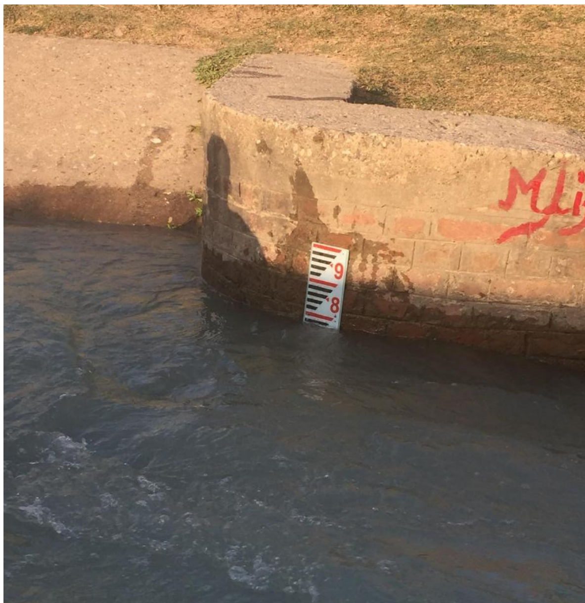
Fig: Installation of Gauge at Flume of Mahendranagar Distributary
