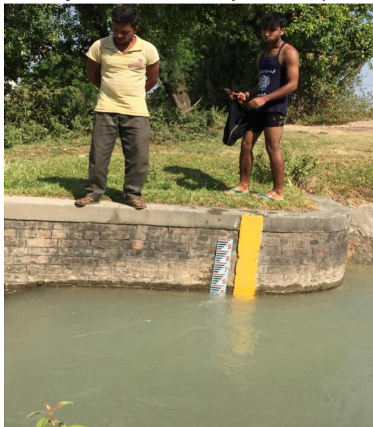
Fig: Installation of Gauge at Flume
